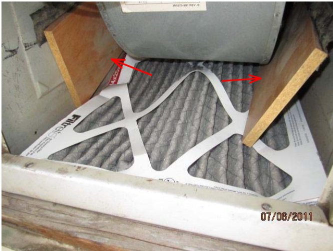
#39 Proper filter hold down straps should be used
