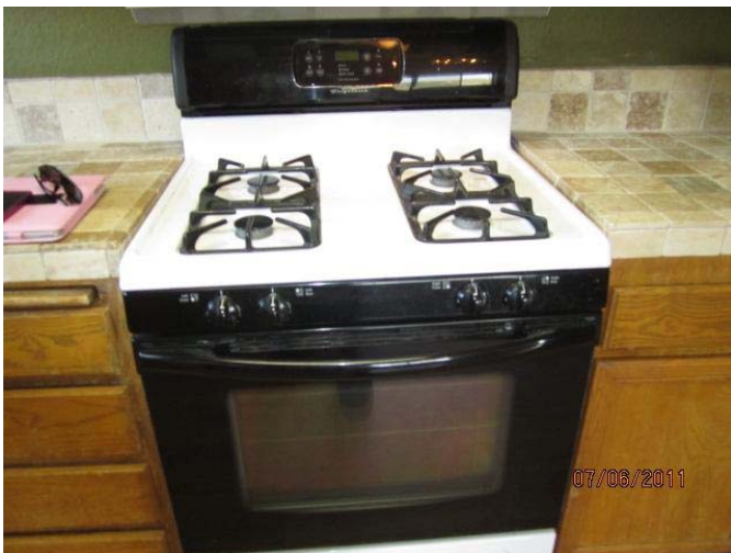
#71 The range is missing the anti-tipping device
