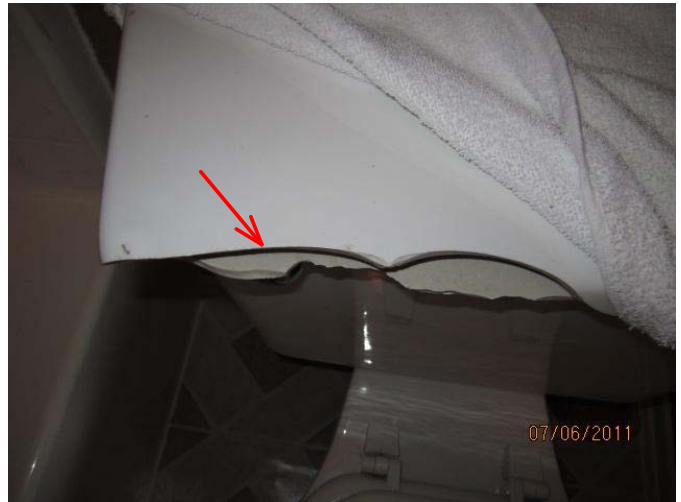
#52 Toilet tank lid is cracked
